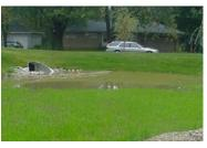
An infiltration basin is a shallow earthen basin constructed in naturally pervious soils and designed for infiltrating stormwater.
