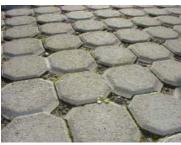
Porous pavement allows stormwater runoff to infiltrate into the ground through voids in the pavement materials.
