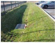
A vegetated swale is a wide, shallow, open channel planted with dense, sod-forming vegetation and designed to accept runoff from adjacent surfaces.
