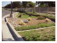
A sand filter is a two-stage constructed treatment system including a pretreatment sedimentation basin and a filtration basin containing sand.
